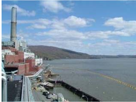
Figure 3-1: Gunderboom® Marine Life Exclusion System™ Deployed at an Existing Intake Structure (Attachment D2)
