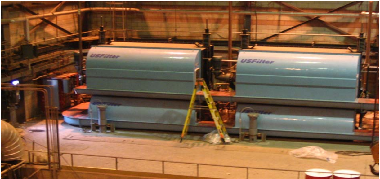
Figure 4-2: Dual Flow Traveling Screen Installation ( www.siemens.com )
