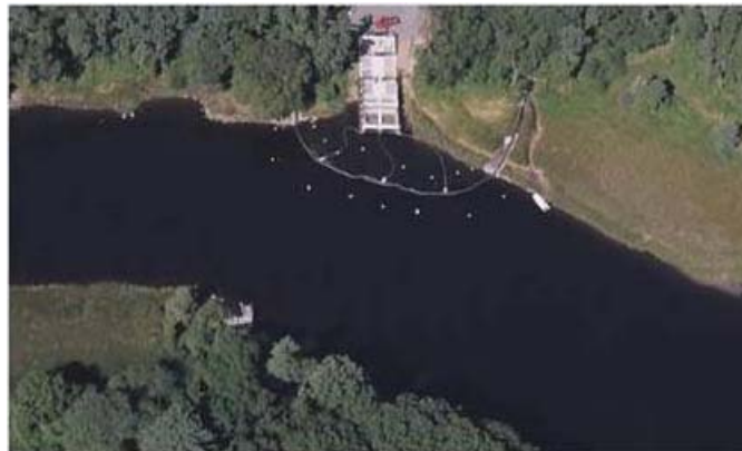
Figure 3-2: Aerial View of a Gunderboom® Marine Life Exclusion System™ Around an Existing Intake Structure (Attachment D2)
